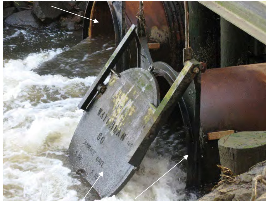
Tide Gate & Culvert in Good Condition
