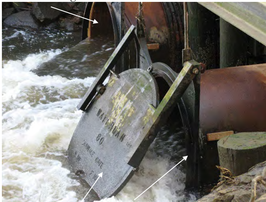
Tide Gate & Culvert in Good Condition
