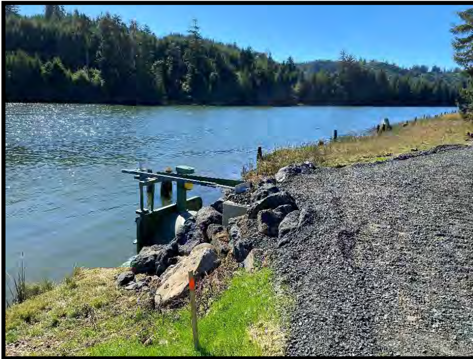
September 2023 – Single tide gate and culvert installation.
